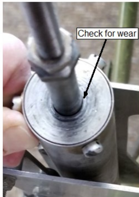
Figure 5. Spring Capsule Wear Inspection Area
