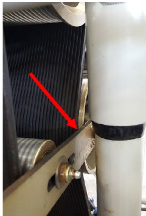
Inspection point – Center pulley, aft edge
