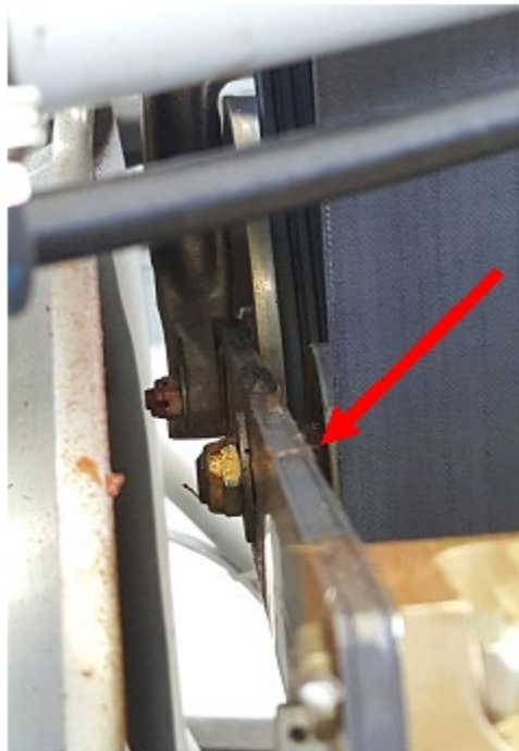
Inspection point – Center pulley, forward edge
