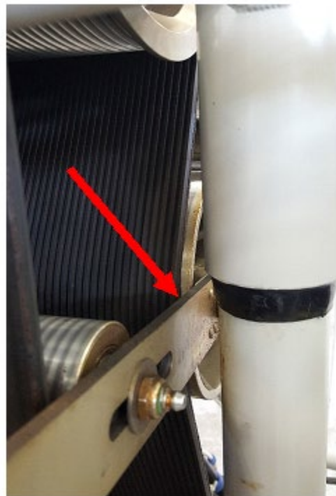
Inspection point – Center pulley, aft edge
