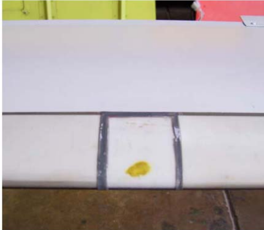
Figure 3. Sealant Applied to Blade Tape Repair Edges
