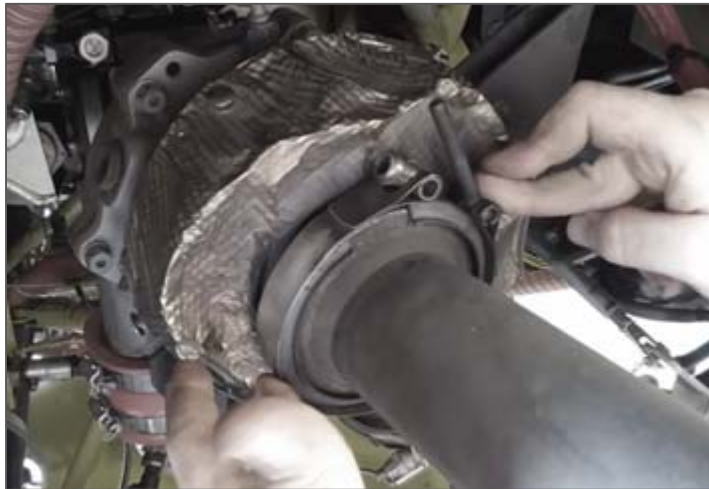
Figure 5c. Flanges and metal gasket joined; clamp positioned over joint
