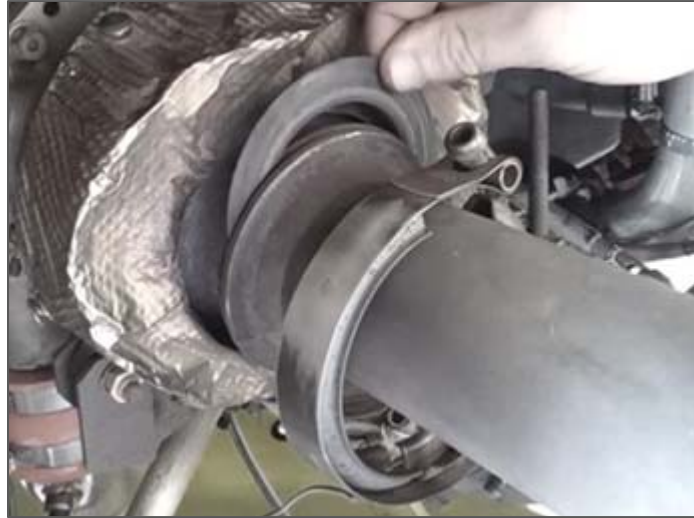
Figure 5b. Installing metal gasket, P/N LW-14485
