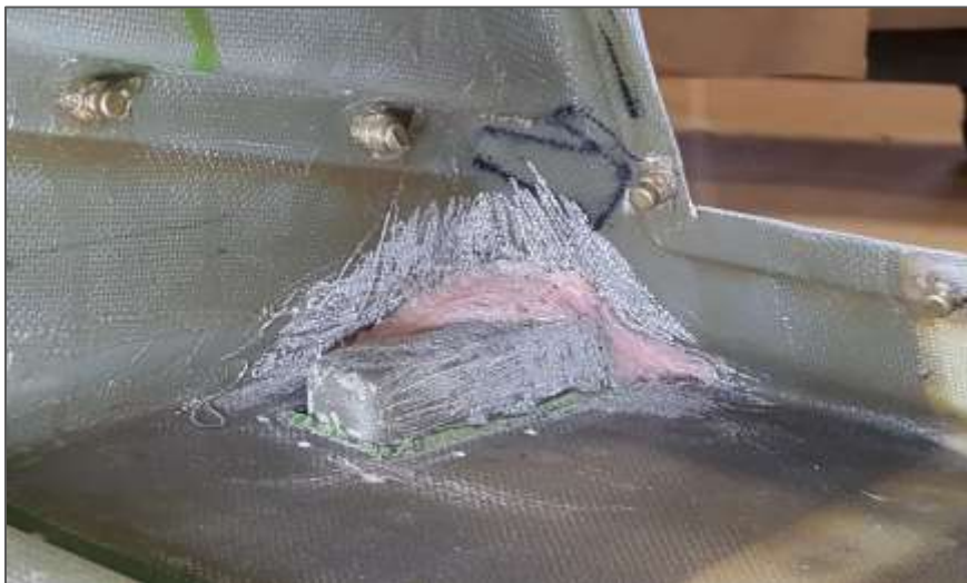
Figure 3. Inside corner hand hold and material (prepared for fiberglass)
