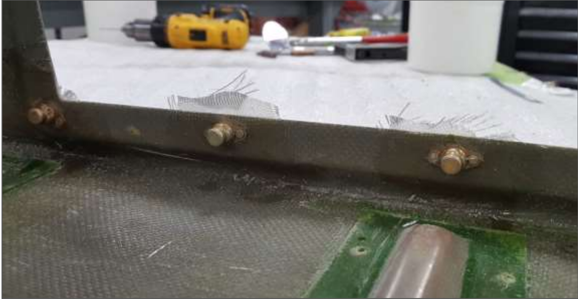
Figure 11. FR 7704-00 polyester resin applied to fiberglass patch
