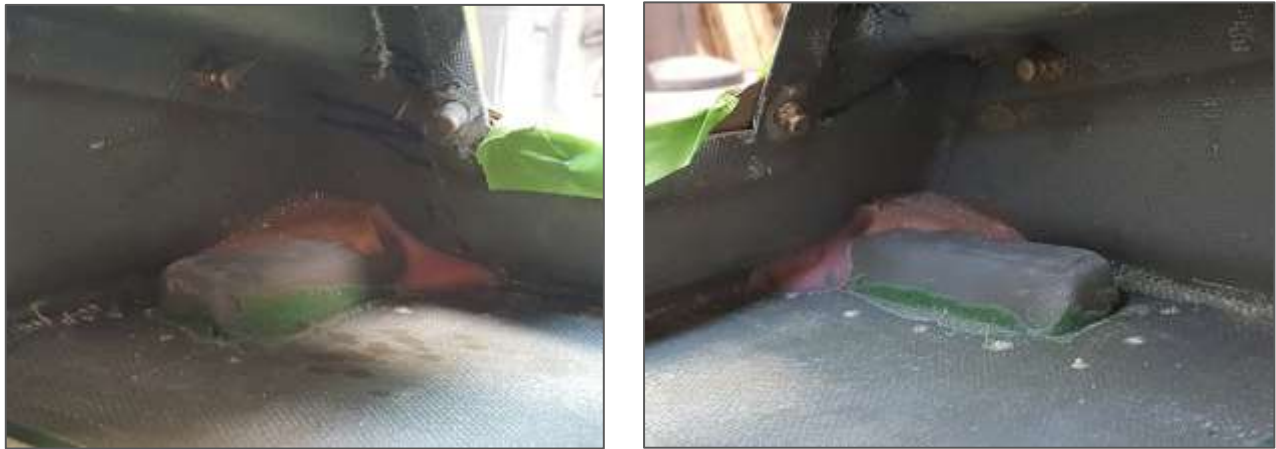
Figure 2. Inside corner hand holds (prior to preparation)
