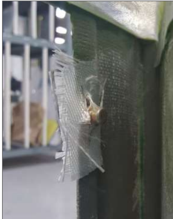
Figure 10. Fiberglass patch applied to nutplate
