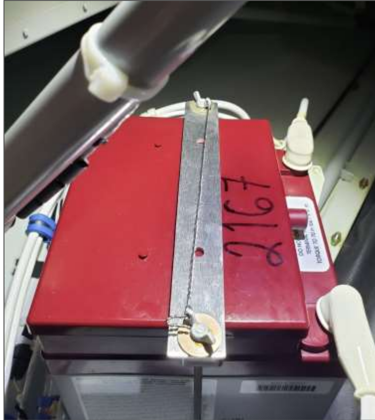
Figure 3. Battery hold down installed
