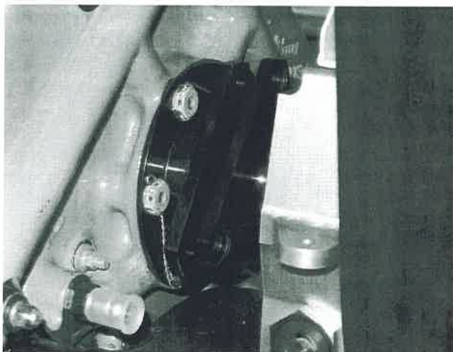
Figure 5 - Engine to Lower Pulley Alignment (Engine Low)
